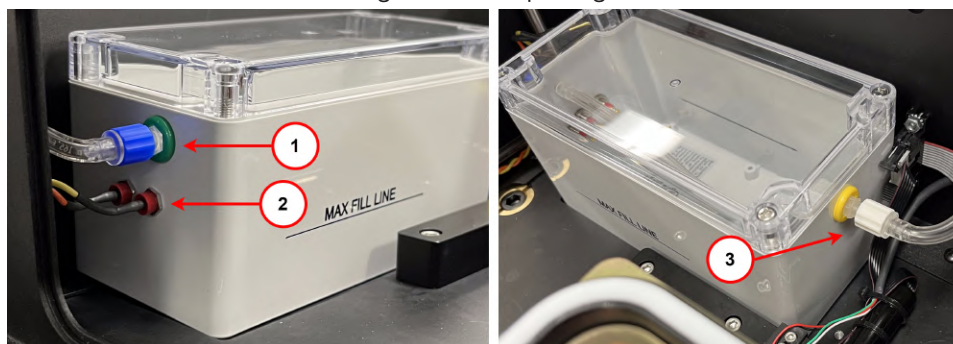
Figure 7-27: Water Reservoir through the Right Side Upper Access Door and Top Door
