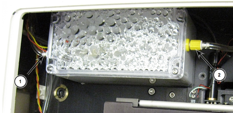
Figure 7-23: CO 2 Tubing Connections on the Water Reservoir
